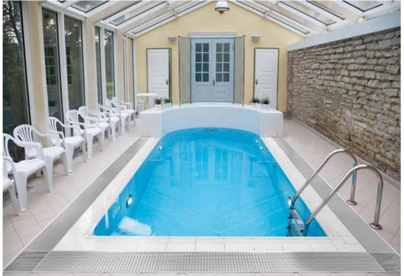
Platinum Grate around perimeter of pool
