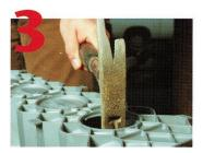
Knockout channel base for outlet at required position
