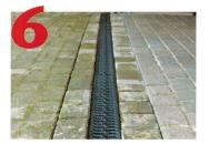
Finish pavement/pavers must be 1/8" higher than the grate.
