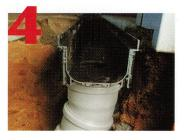
Push-fit outlet adapter into bottom of channel, lay outlet channel first and connect 3" or 4" SDR pipe or 4" schedule 40.
