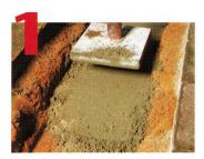
Excavate area to accomodate trench drain and 4" concrete surround, compact base.
