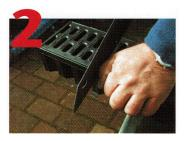
Cutchannels to fit required length (if necessary)
