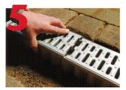
Lay 4" deep concrete bed. Lay channels working away from outlet, channels slide-fit together. Make sure to keep grate top inside trench while filling to avoid squeezing trench
